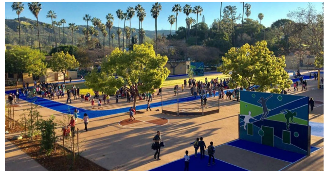
EAGLE ROCK ELEMENTARY SCHOOL, IN LOS ANGELES, CA, REMOVED 23,789 SQUARE FEET OF ASPHALT, REPLACING IT WITH PERMEABLE SURFACE AND NATIVE/DROUGHT TOLERANT TREES AND PLANTS, CAPTURING EXCESS RAINWATER.
