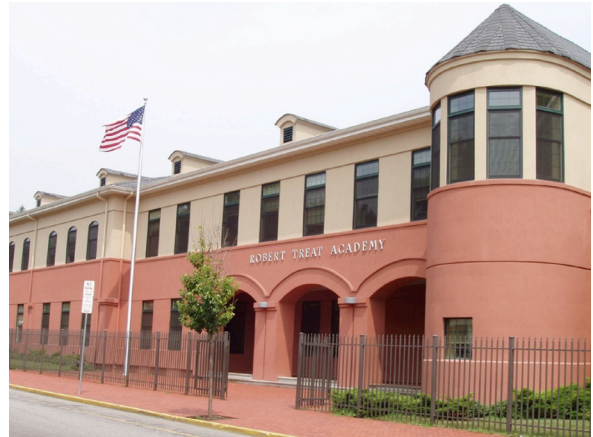
RTA was built from the ground up.
