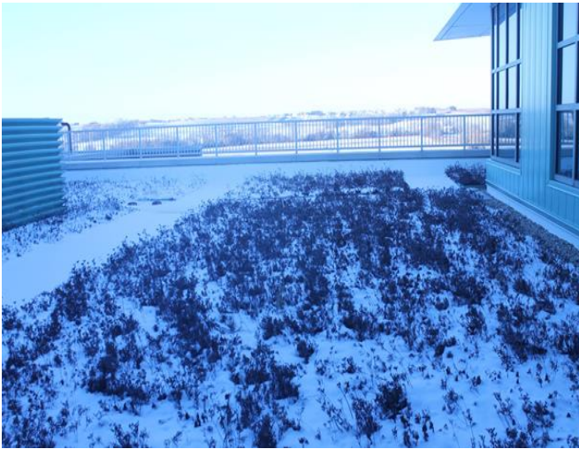
One of two green roofs used to redirect sunlight.
