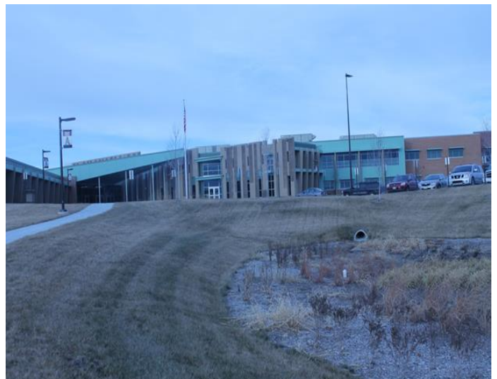
Retention pond between the parking lot and the building.
